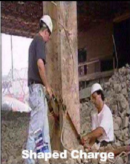
This show demolition chargers being placed on a steel column. Notice the angle of the charge. This is done to cause the building to slide or jump and collapse into it's footprint
